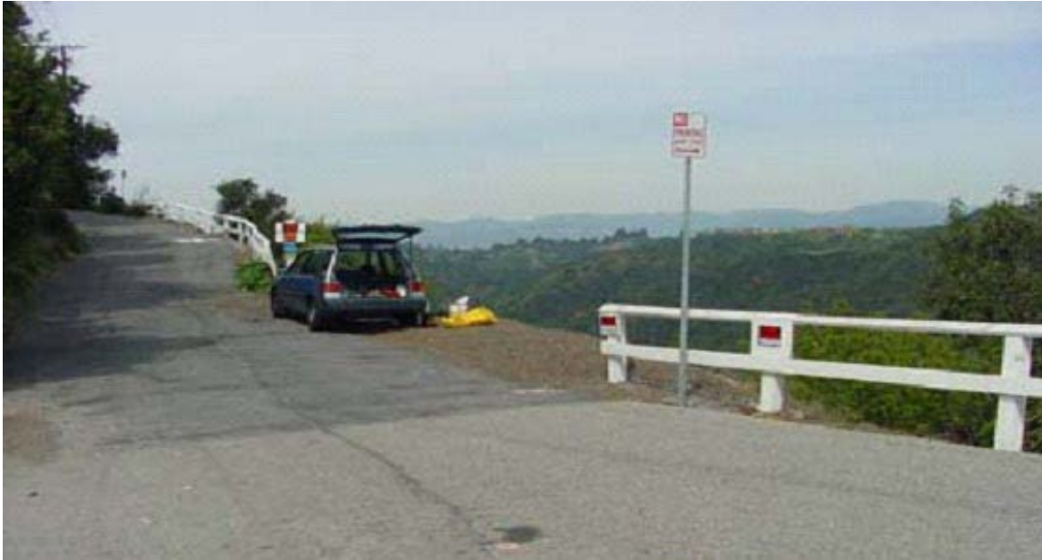
Photo 1. Citizen complainant's property before the wall was constructed.
