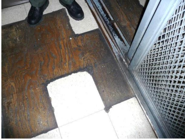
Detainee elevator floor is missing sections and is uneven and worn. Portions of broken tile could be used as a potential weapon.
