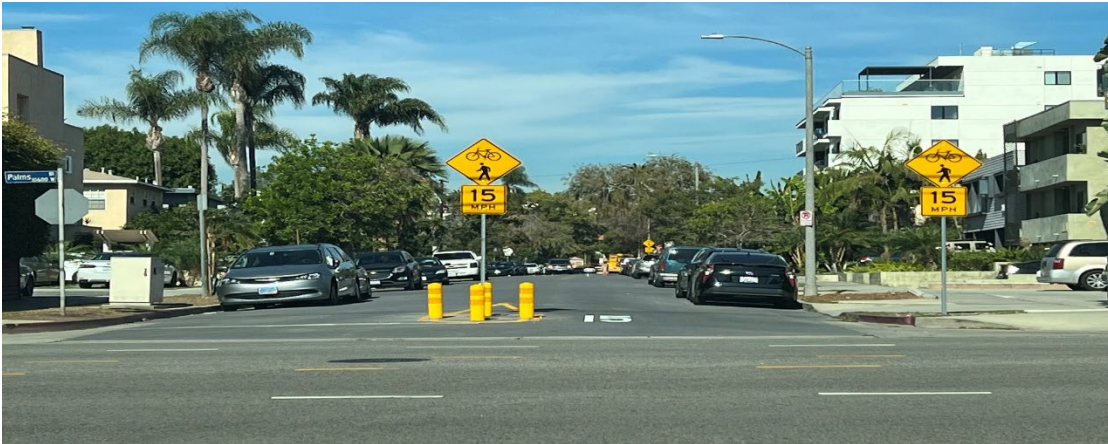
Photo 29 Another approach to significantly lower traffic speeds through lane restriction, width reduction, and signage while including warnings to watch for cyclists and pedestrians
